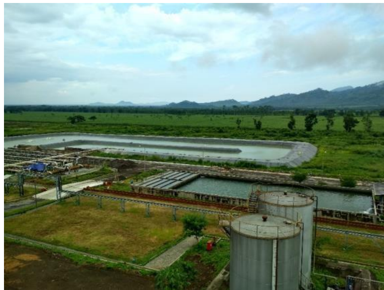
Gambar 3.7 Bagian Water Treatment Plant
