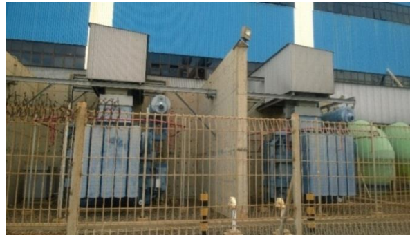
Gambar 3.43 Auxiliary Transformer
