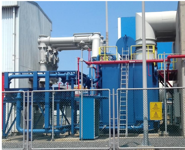
Gambar 4. 1 Generator Transformer 765 MVA
