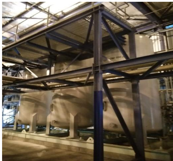
3.3.5 Demineralizer Gambar 3.20 Mixed Bed
