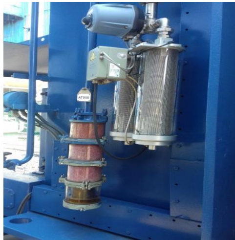
Gambar 4. 8 Dehydrating Breather
