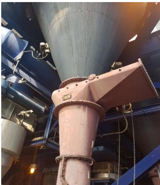
Gambar 3.9 Gambar Coal Silo
