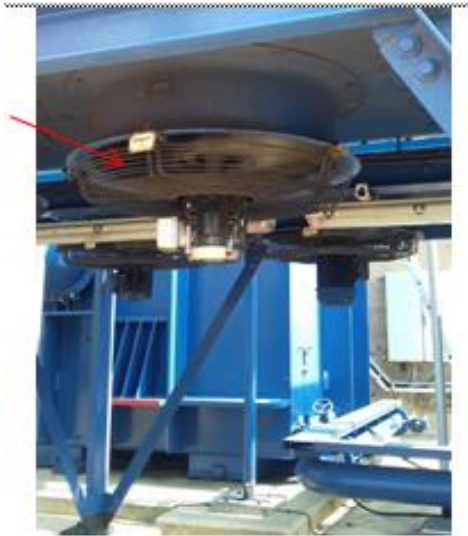
Gambar 4. 5 Cooling Fans
