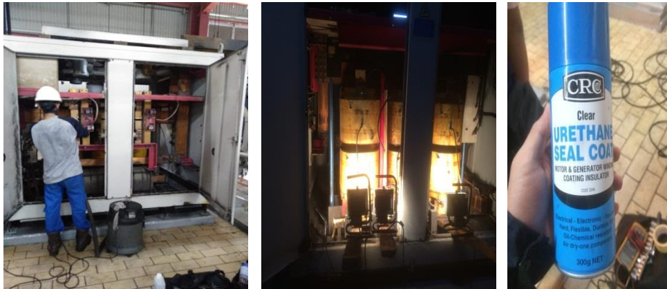
Gambar 5. 5 Maintance Transformer
