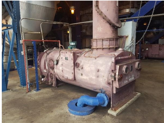
Gambar 3.10 Coal Feeder
