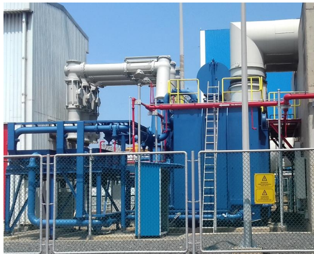
Gambar 5. 1 Wet Transformer (step up) BAT01
