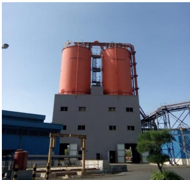
Gambar 3.36 Fly Ash Silo
