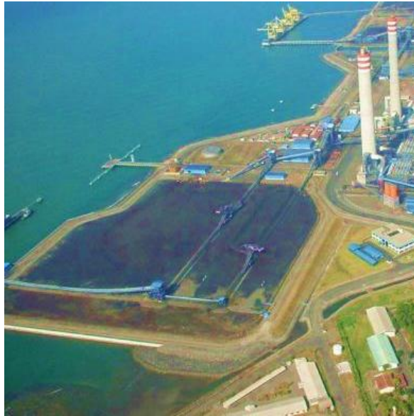
Gambar 3.7 Coal Plant PLTU PT. YTL Unit 5 & 6
