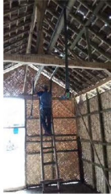
Figure 3. water pump installation
