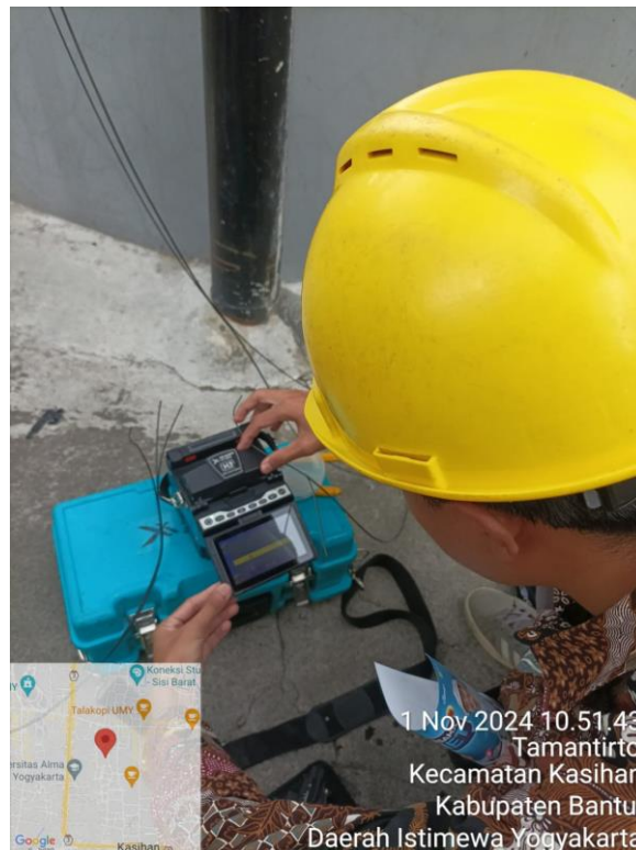
Gambar 4. 20 Proses Splicing
