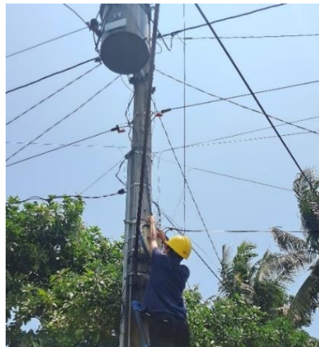
Gambar 3. 6 Perapian Kabel KU serta Dropcore
