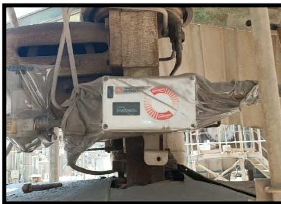
Gambar 40. Positioner Control Valve
