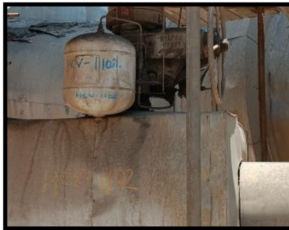
Gambar 39. HCV ( Hydraulic Control Valve )
