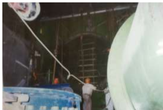
Gambar 4. 7 Water Box (Sumber : PT POMI)
