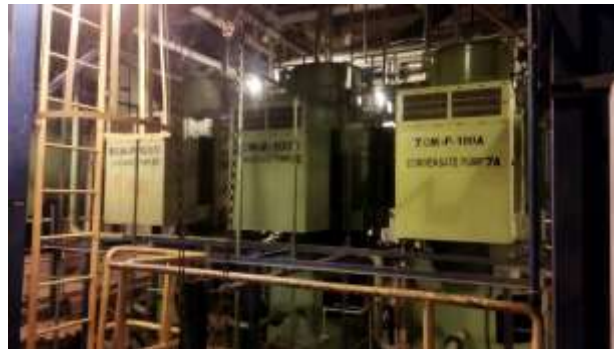
Gambar 4. 11 Condensate Extraction Pump
