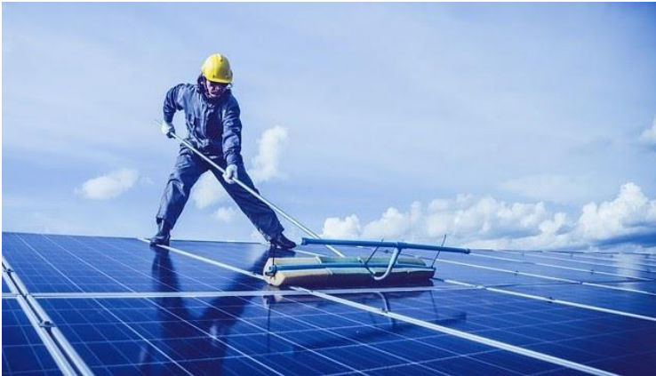
Gambar 3.5 Cleaning PV
