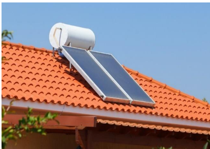
Gambar 3.5 Solar Water Heaters
