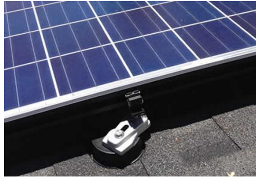
Gambar 4.20 pemasangan model rail less (Sumber: Sanspower.co.id )
