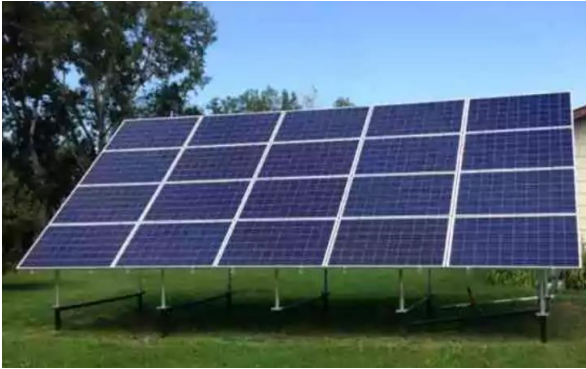
Gambar 5.4 Pemasangan Jenis Ground Mount (Sumber: pasangpanelsurya.com)
