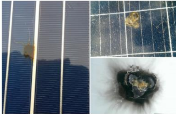
Gambar 5.15 Panel Surya Terbakar (Sumber: ica solar)
