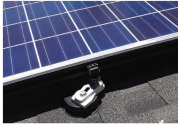
Gambar 4.20 pemasangan model rail less (Sumber: Sanspower.co.id)
