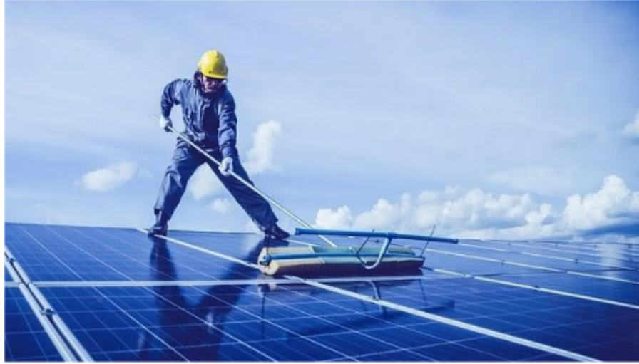
Gambar 3.5 Cleaning PV
