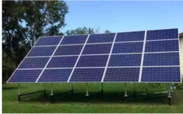
Gambar 5.4 Pemasangan Jenis Ground Mount (Sumber: pasangpanelsurya.com)
