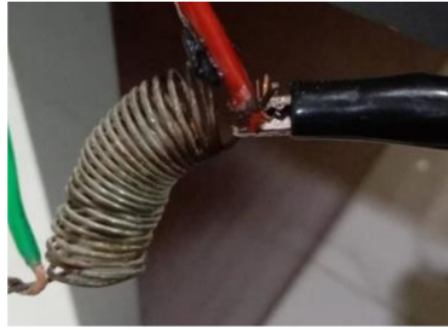
Figure 4. The heater coil mounted on the pipe.
