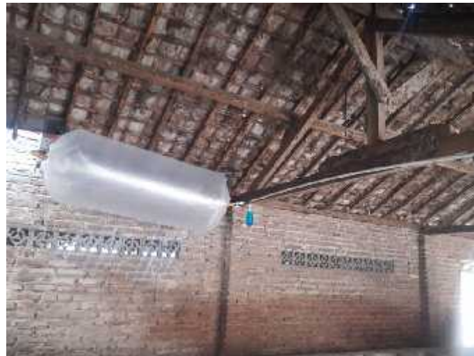
Figure 6. Gas pipelines and gas container
