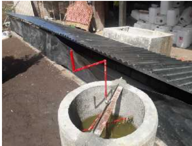
Figure 3. Inlet chamber
