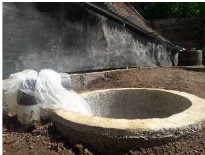
Figure 5. Outlet chamber
