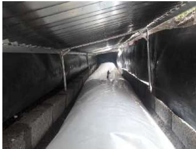
Figure 4. Balloon digester
