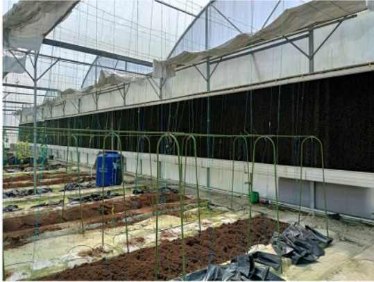
Fig. 17 Installation of a cooling deck system
