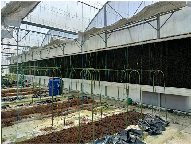
Fig. 17 Installation of a cooling deck system
