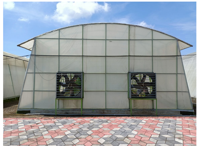
Fig. 20 Exhaust fan for effective circulation of the air in the smart green house
