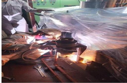
Gambar 3. 1 Pemasangan Water Separator/diesel
